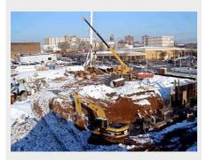
As a result of a 15 feet high historic retaining wall that could not be disturbed, Whitestone developed an economical foundation solution involving two foundation systems for this student housing center in Newark, NJ. Whitestone also conducted environmental and geotechnical due diligence investigations in support of the proposed redevelopment project and managed environmental remediation efforts for this Brownfield redevelopment. Read More...
